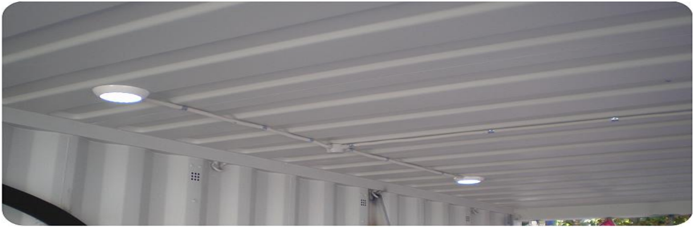
Container with two LED dome lights, Optional flexible conduit and junction box was included to run cable along roof
